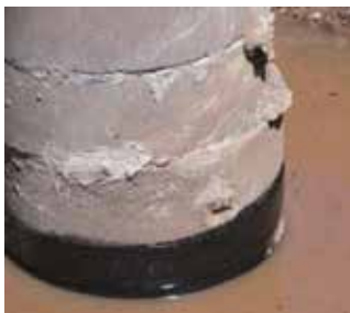
RISER-WRAP® used to rehab an existing manhole submerged in runoff water.
